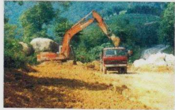
Photo 10 : The emergency clearing work at the site
