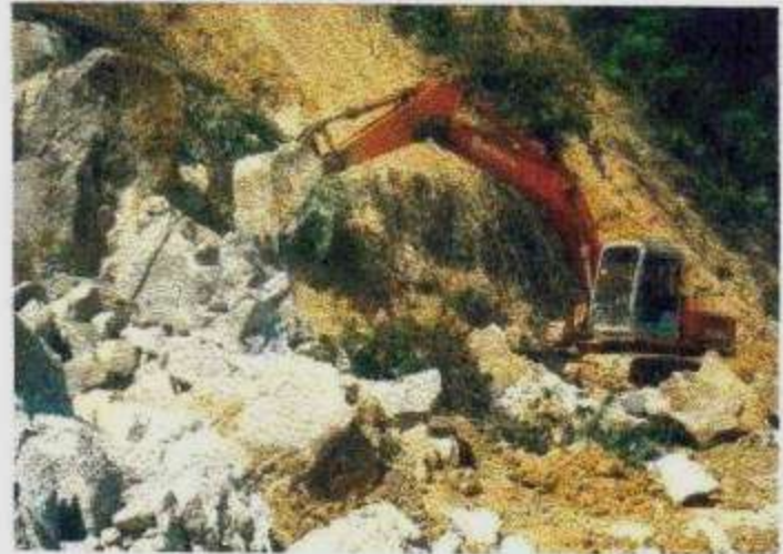
Photo 14 : The boulders clearing work
